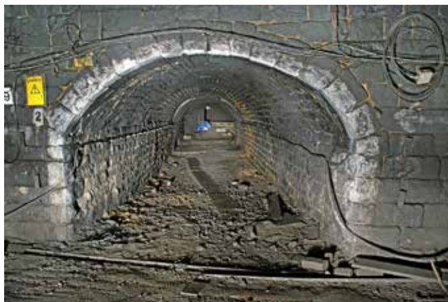
One of the cross tunnels. Photo Mitch Preston
